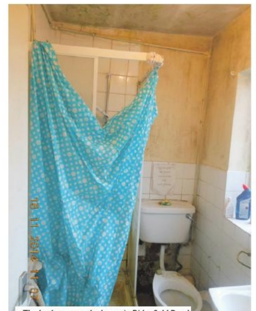
• The bathroom at the house in Ridgefield Road
